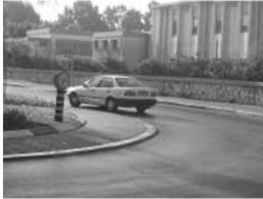
Figure 4. A roundabout that functions like a narrow road for small cars but also as a wide road for large vehicles
